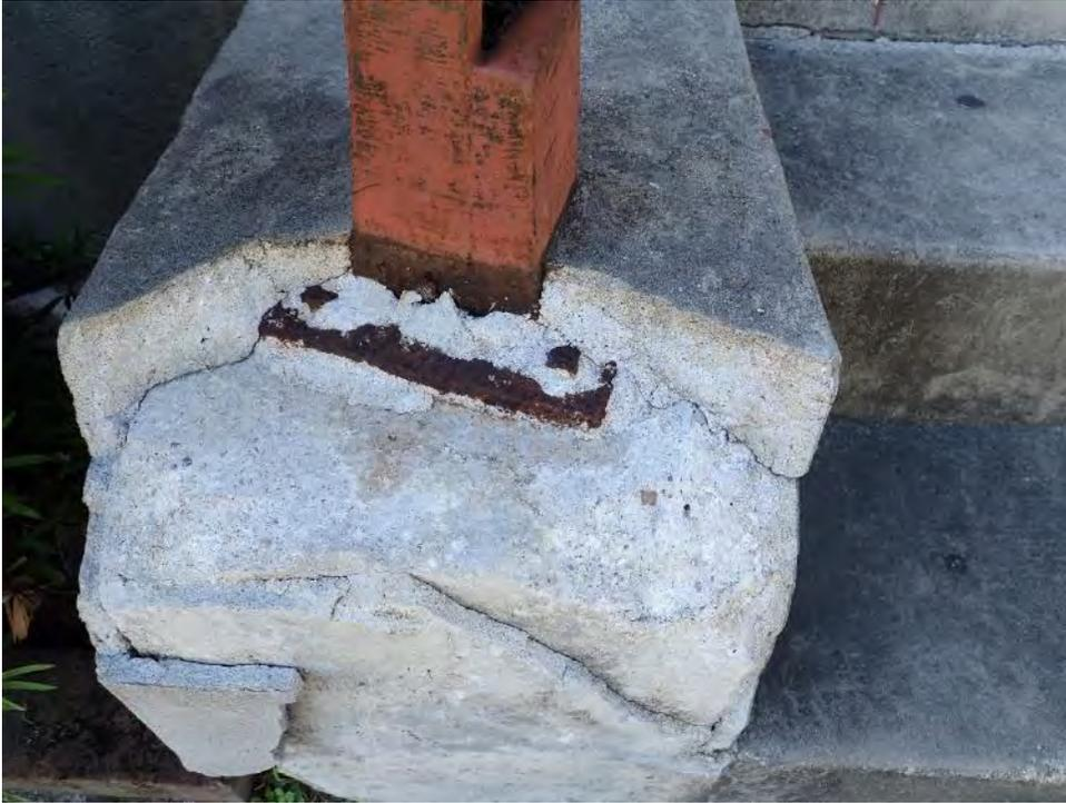
**17** Spalled concrete door stop at Southwest Corner
