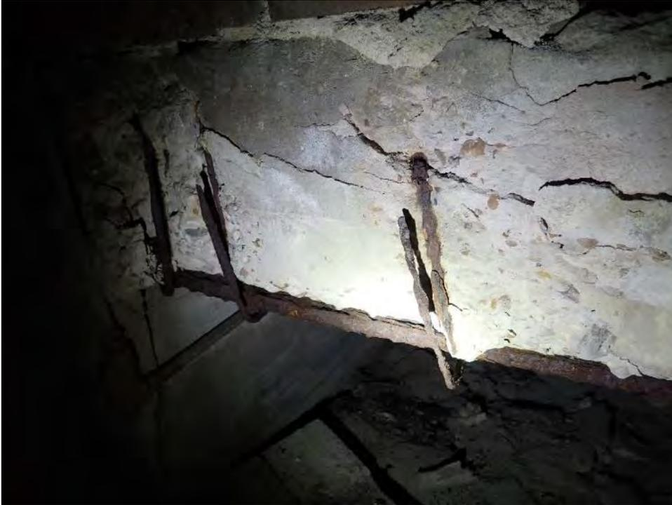
**03** Exposed corroded rebar on back entrance to ventilation shaft
