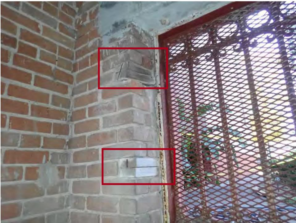
**04** Missing bricks at gate under bearing end of concrete beam
