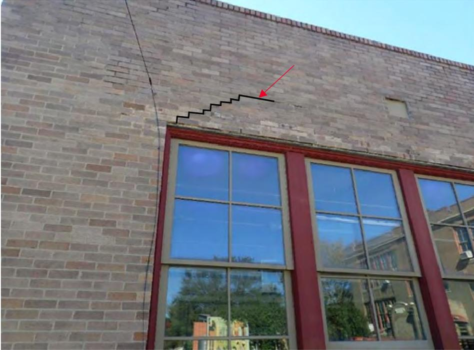
19 Stair step cracking
