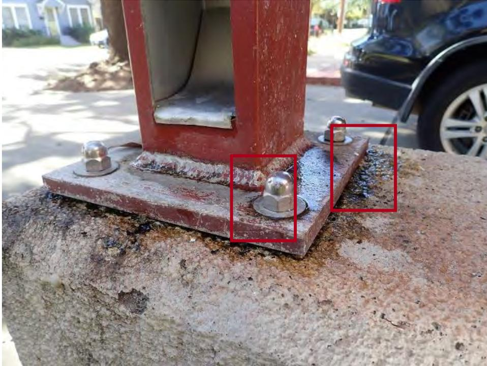
25 Latent moisture and corrosion at base of column
