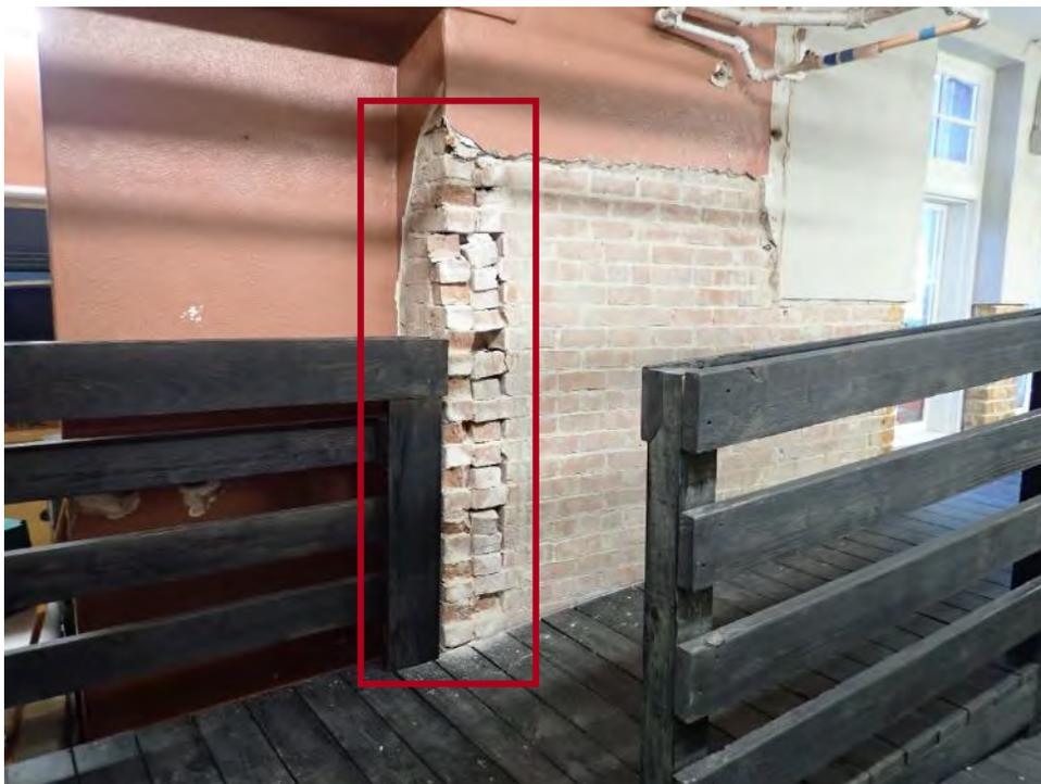
06 Loose and missing bricks in an intersecting brick wall
