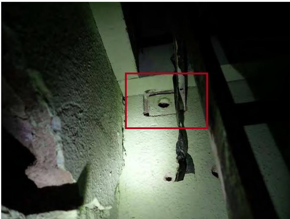
22 Missing roof access ladder support
