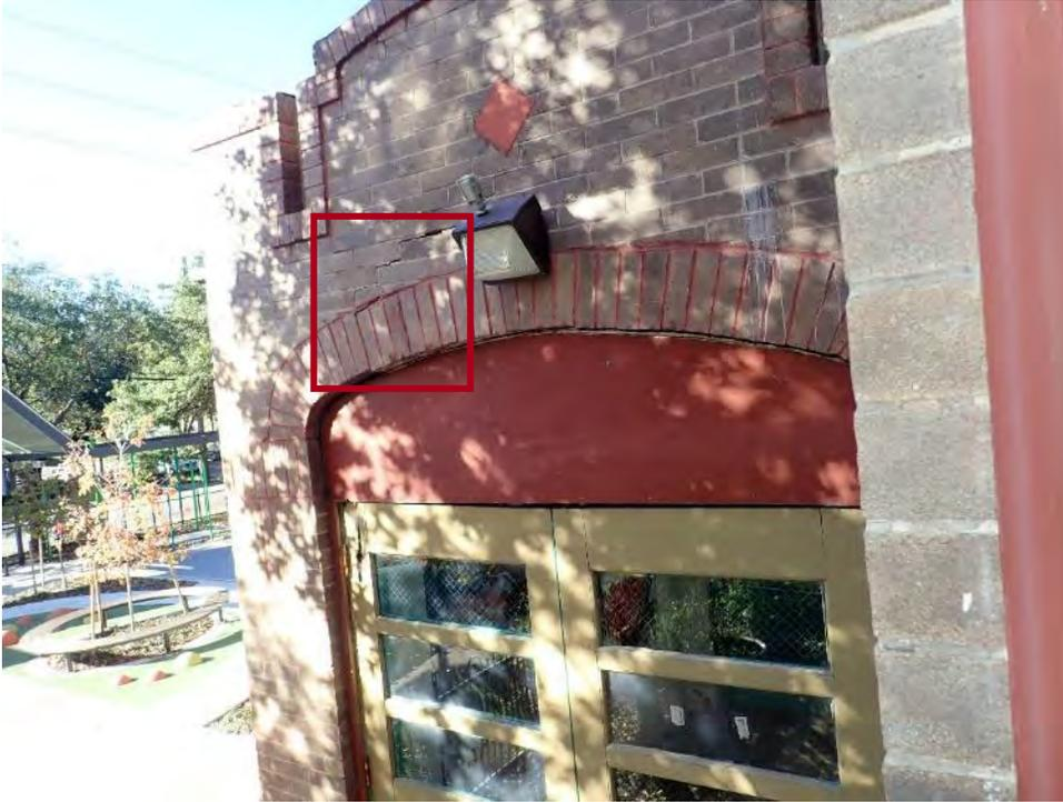
**11** Stair step cracking above the arch
