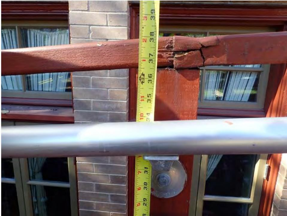
15 Deteriorated wood handrail at East Entrance3
