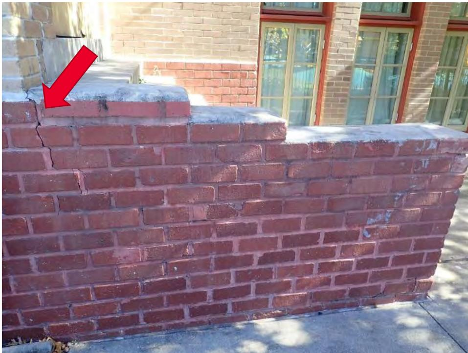
10 Stairstep cracking in exterior wall
