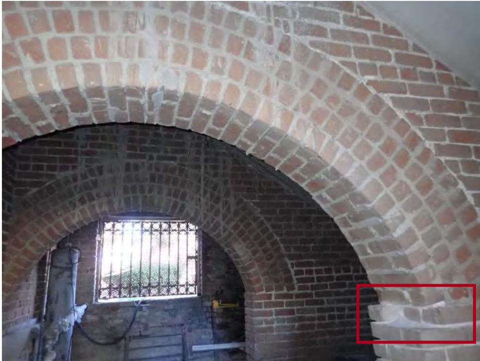
05 Missing bricks and severely deteriorated mortar at the springpoint
