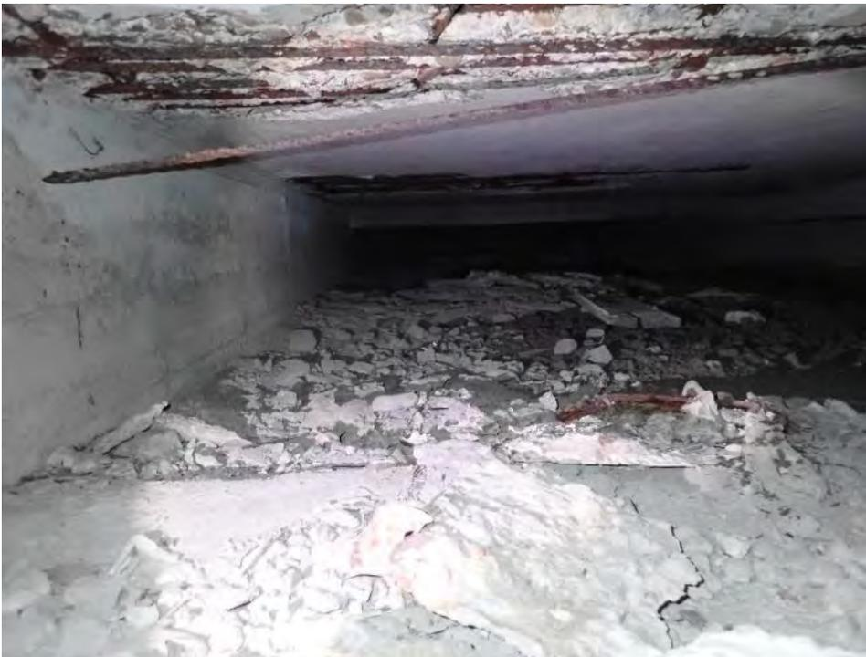
**02** Exposed, corroded bars and fallen concrete in ventilation shaft under slab
