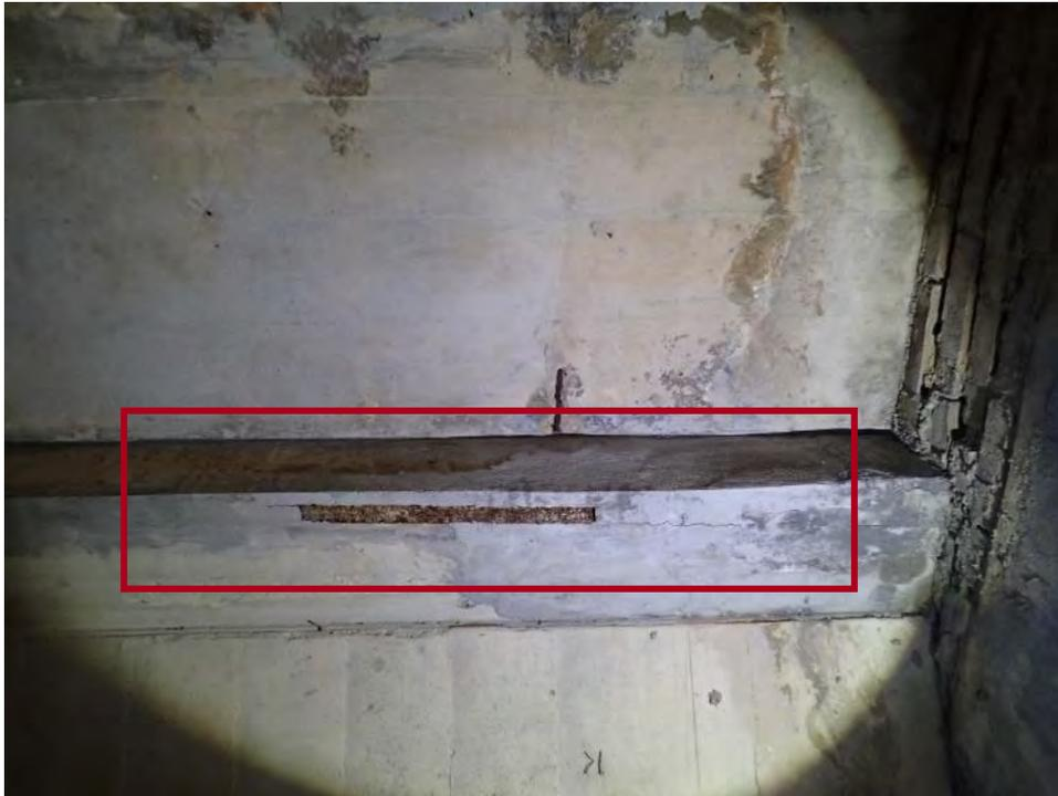
**07** Spalling overhead slab under main entrance
