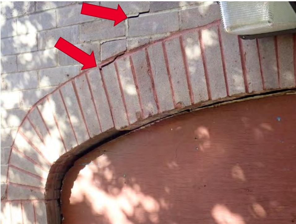
**12** Close-up view of the cracking and dislodged brick at west entrance
