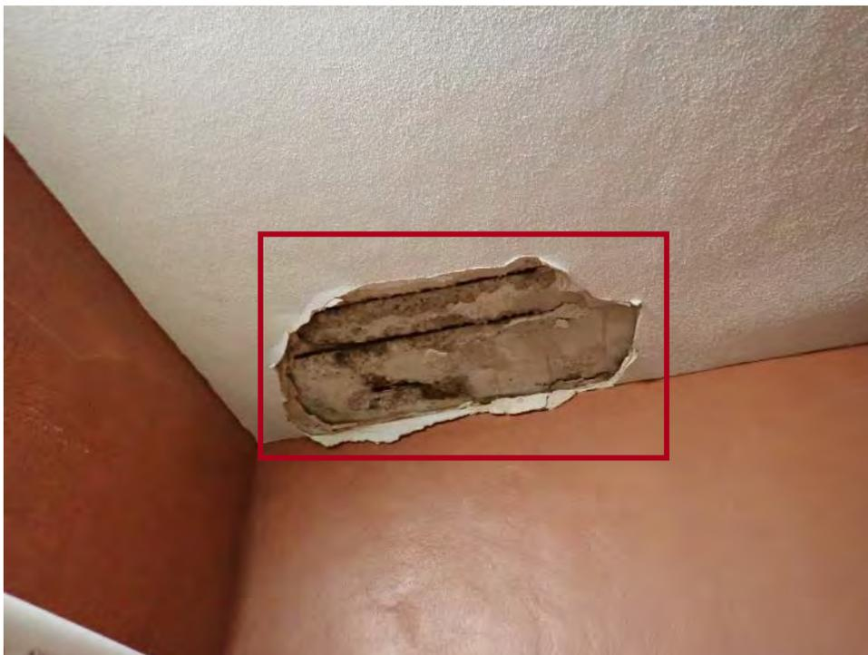
**08** Overhead spall in the interior storage room under the main entrance
