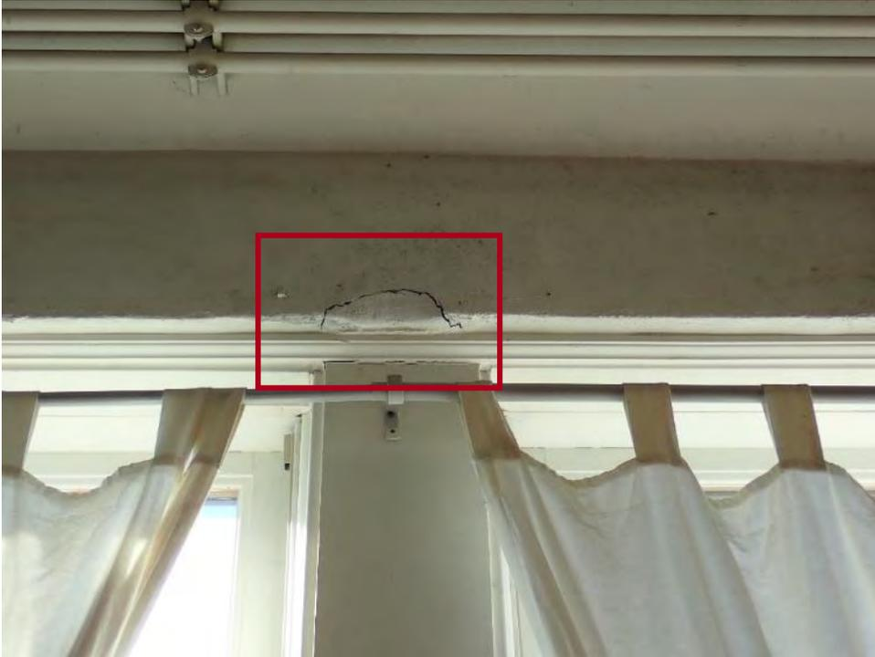
27 Spall above window on 3<sup>rd</sup> floor (Typical)
