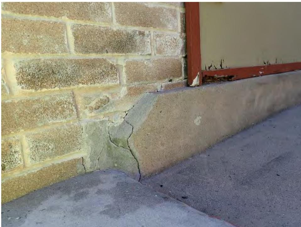
16 Spalling curb on North side of East Entrance
