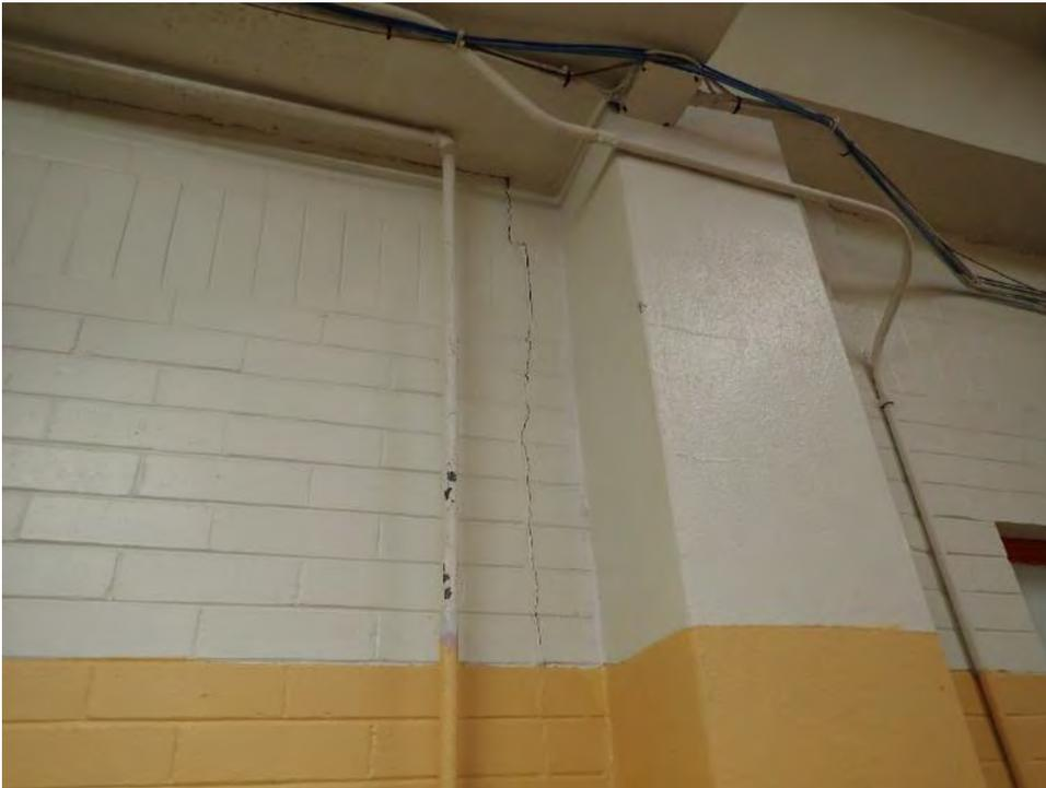
20 Cracking at transition between original building and extended East Wing
