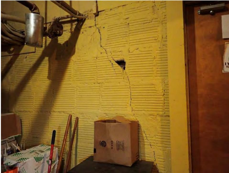
21 Cracking of clay infill tiles
