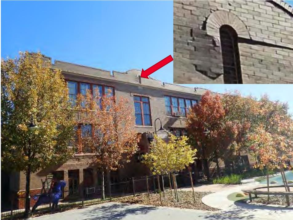
09 West elevation, the area with bulged bricks is enlarged
