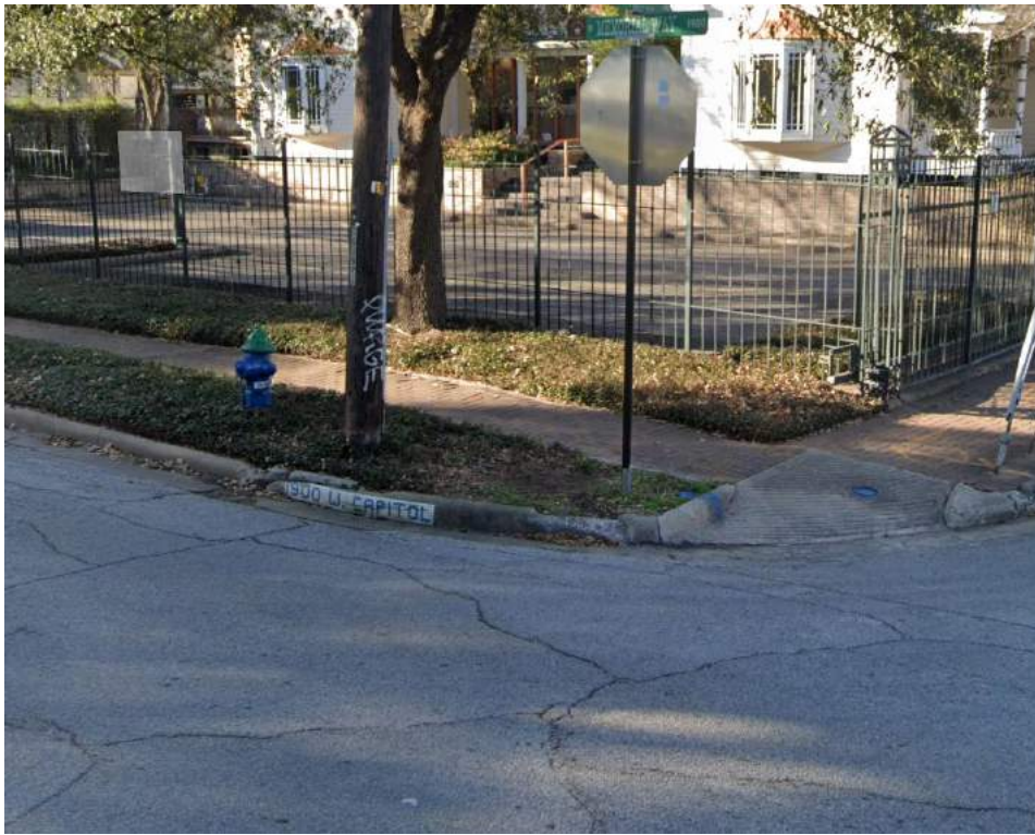
North Memorial Way/W. Capitol before Construction
